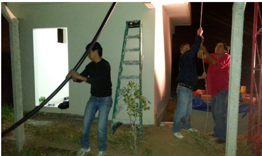
Engineers working late into the night to finish the installation of antennas getting ready for inspection in two days.
