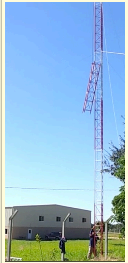
Erecting the new tower
