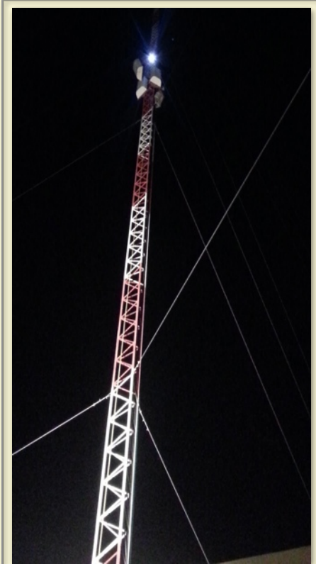
Installation of antennas prior to government inspection.
